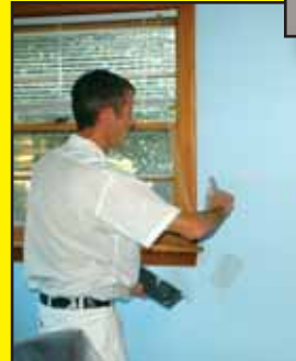
Pat Kukosh patched water damage in the living room ceiling, repaired holes in bedroom walls, and caulked exterior trim prior to painting.
