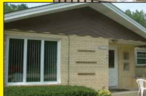
Trim on the front of the house was rejuvenated with fresh coats of brown on the fascia and white on the soffits.
